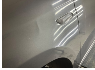
Çamurluk, sol, Çamurluk, sol > Ezik
