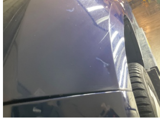
Çamurluk, sol, Çamurluk, sol > Ezik
